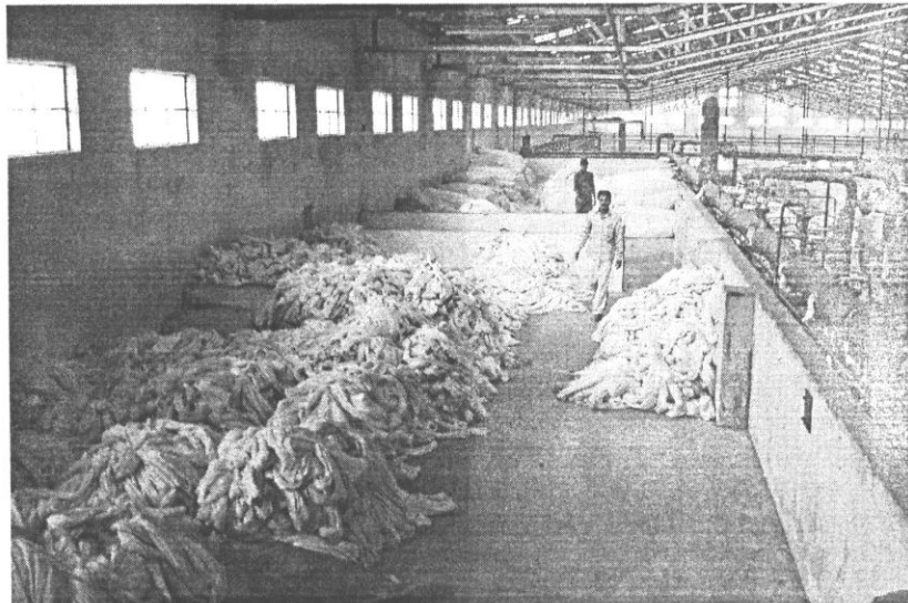
Fig. 10.3 Hazard - No Windows and Closed Ventilators →
