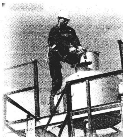
Clean Platform and Safe Method of Working
