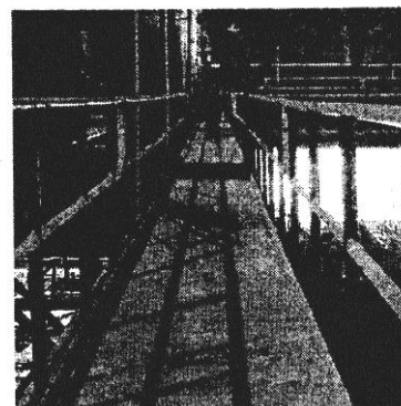
Fig. 7.3 Catwalk, tow guard and railing
